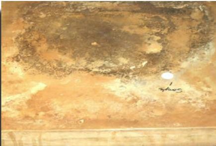
The acid in chemical stains opens the top surface of the concrete, allowing metallic salts to reach the free lime deposits. Water from the stain solution then fuels the reaction, usually for about a month after the stain has been applied.
